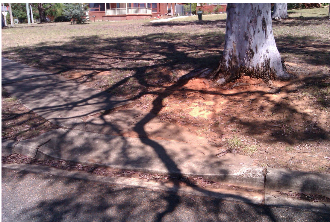
Figure 16(b): High lip, steep ramp and uneven paving present obstacles for path users with wheels and a trip hazards for pedestrians. (Captain Cook Crescent)
