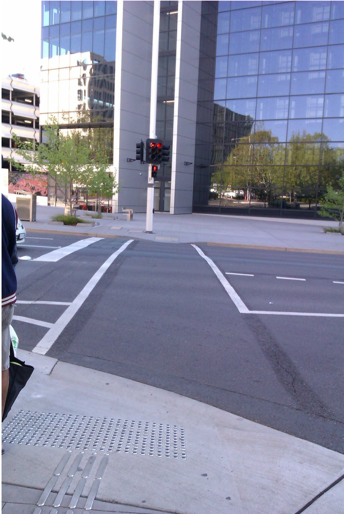
Figure 18(a): Road crossing on northwest side of intersection of Marcus Clarke and Alinga Streets in Civic, showing very narrow ramp on northern side, wider ramp on southern side.
