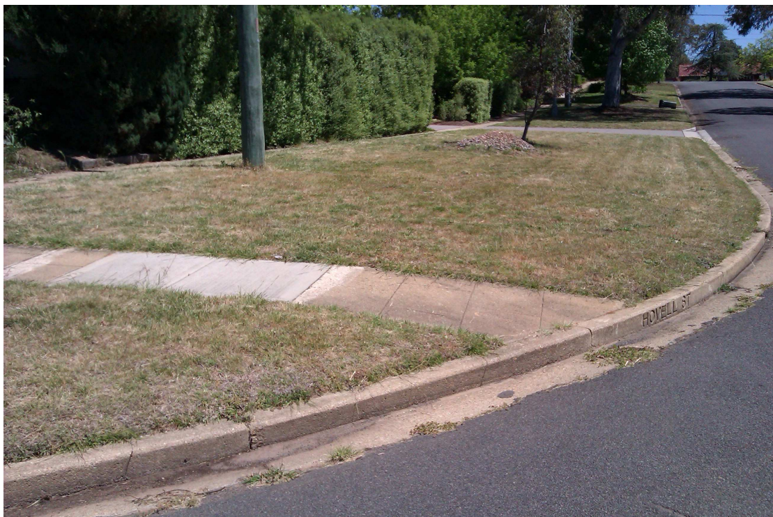
Figure 15: Path without ramp to road. The difficulty traversing this step deters pram users from using the path – and, if they do, they spend longer crossing the road as they manoeuvre the pram up or down over the kerb. This obstacle is impossible for most cyclists to traverse. (Corner of Hovell Street and Meehan Garden, Griffith)
