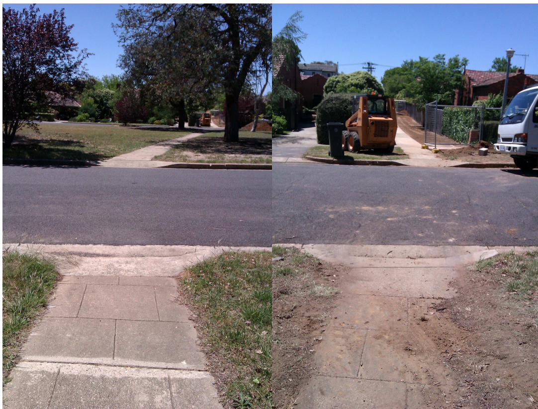
Figure 17: Path ramps to roads vary in gradient. Only the one in the bottom left of the pictures above is user-friendly. (Meehan Gardens)
