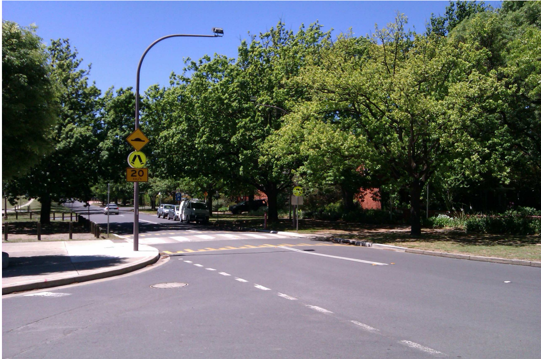
Figure 19: This pedestrian crossing is given clear priority over road users and is seamless with paths on either side of the road. (Throsby Crescent, Griffith)
