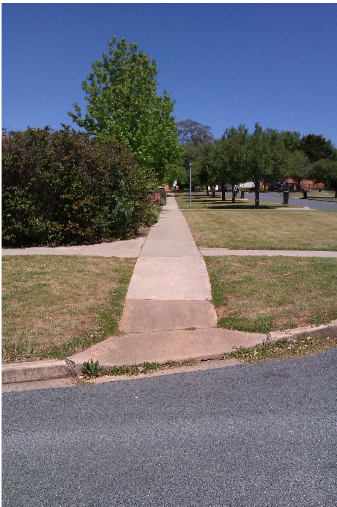
Figure 16(a): High lip where ramp meets road provides an obstacle for path users with wheels (which means they spend longer on the road as they try to get over the lip) and a trip hazard for pedestrians. Steep section between ramp and main pathway compounds the problem. (Wild Street and Walker Crescent intersection, Narrabundah)
